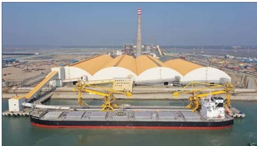
A view of Matarbari coal power plant
