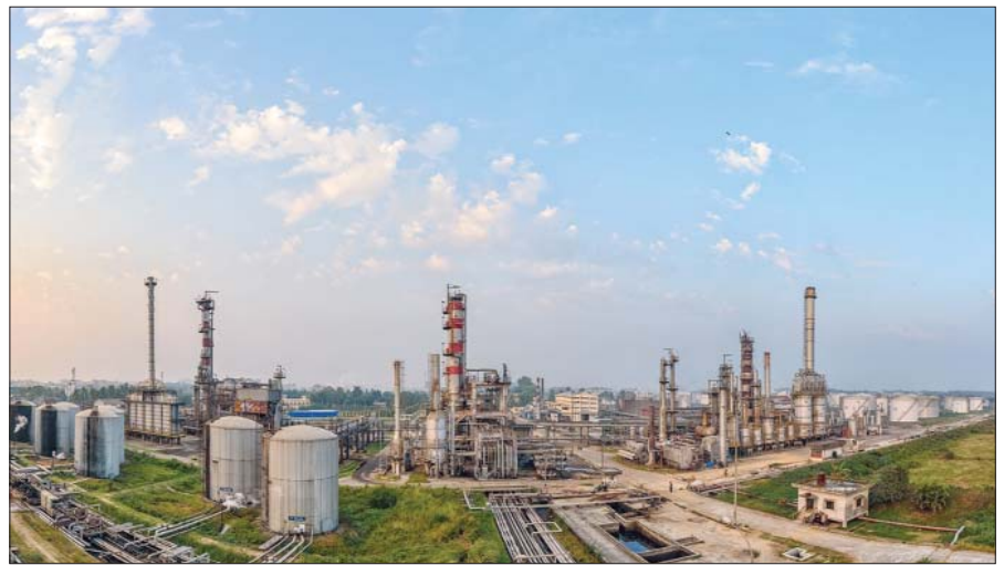
A view of Eastern Refinery Limited
